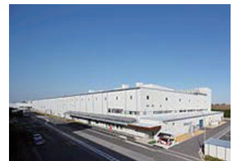
The waterborne paint Plant
