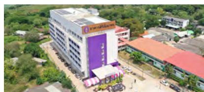
Hospital with a rooftop solar power system installed as part of the "Solar for Lives" environmental project
