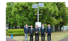
Launch of a demonstration project for autonomous street lighting in cooperation with the city of Okazaki, Aichi Prefecture (April 2023)
