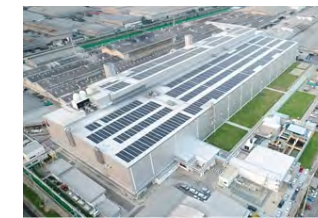
New paint plant (MTh)
