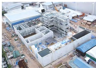
Discharged water recycling plant under construction (Thailand)
