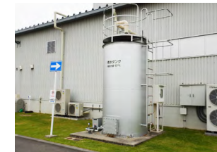
Rainwater storage tanks (Okazaki Plant)
