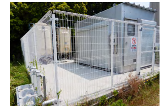
Groundwater membrane filtration equipment (Okazaki Plant)
