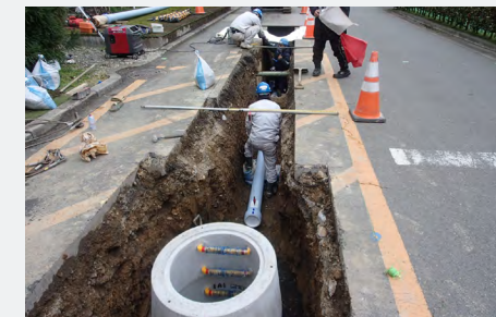
Underground construction to install wastewater piping for factory water discharge (Kyoto Plant)
