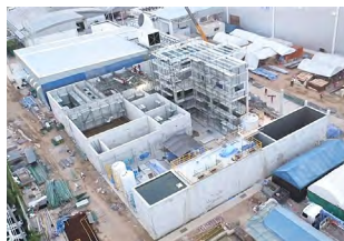
Discharged water recycling plant under construction (Thailand)
