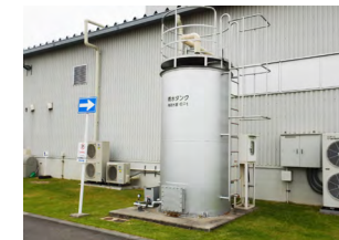
Rainwater storage tanks (Okazaki Plant)
