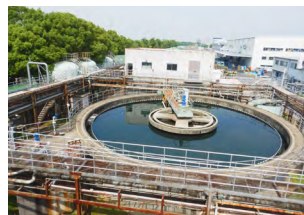
General effluent treatment facilities (Okazaki Plant)
