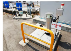
Surface oil detector (Okazaki Plant)
