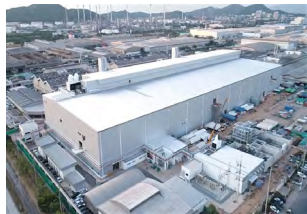
New paint plant under construction in Thailand (MMTh)
