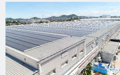
Large-scale rooftop solar power system that commenced operation at MMTh
