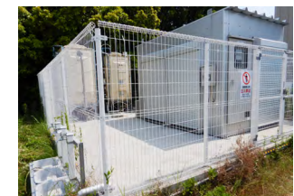
Groundwater membrane filtration equipment (Okazaki Plant)
