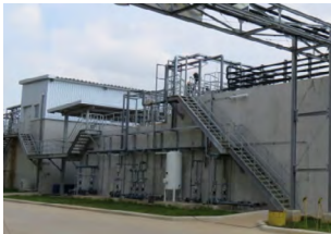
Industrial water and wastewater treatment plant (Indonesia)
