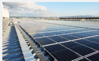
Large-scale solar power plant
