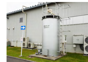
Rainwater storage tanks (Okazaki Plant)
