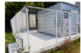
Groundwater membrane filtration equipment (Okazaki Plant)
