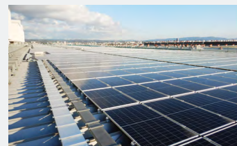
Large-scale solar power plant
