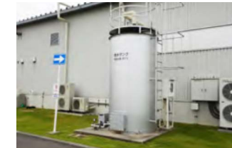
Rainwater storage tank (Okazaki Plant)
