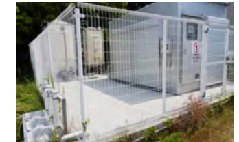
Groundwater membrane filtration equipment (Okazaki Plant)
