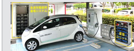
Demonstration facility for utilizing used batteries
