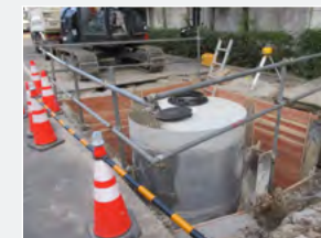
Manhole-type oil-water separator installed in the storm drainage path
