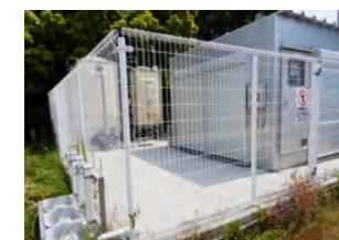
Groundwater membrane filtration equipment (Okazaki Plant)
