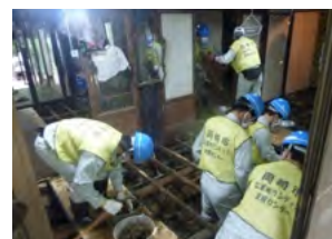
Removing mud from under the floor
