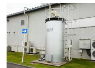
Rainwater storage tanks (Okazaki Plant)
