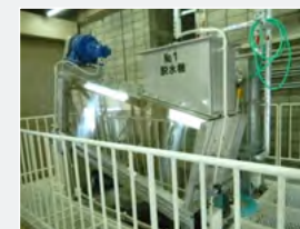
Newly installed screw-type sludge dewatering equipment
