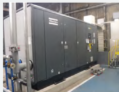
Upgraded inverter-type compressor
