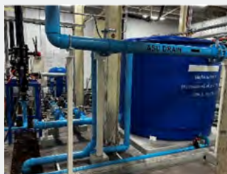
Installed condensate water storage tank
