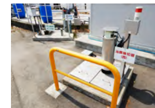
Surface oil detector (Okazaki Plant)
