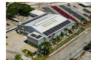
Solar panels erected on the roof of MMPC's plant
