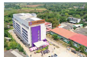
Hospital with a rooftop solar power system installed as part of the "Solar for Lives" environmental project
