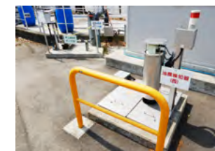
Surface oil detector (Okazaki Plant)
