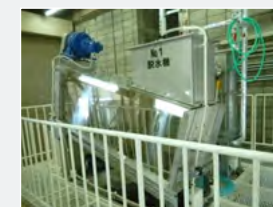
Newly installed screw-type sludge dewatering equipment
