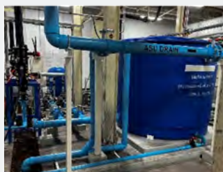
Installed condensate water storage tank
