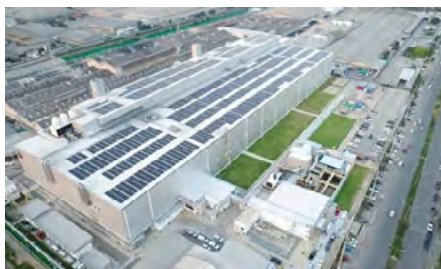
Paint plant (MMTh)
