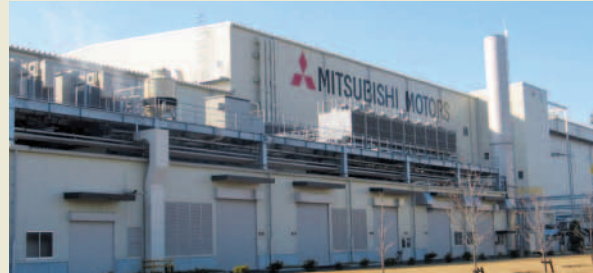
New paint shop (Mizushima Plant)
