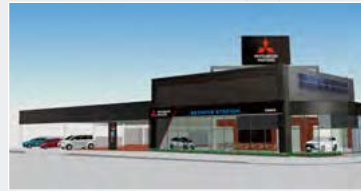
Accelerating the deployment of Dendo Drive Stations
