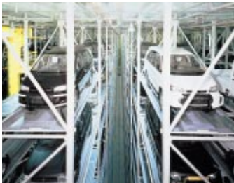
Automatic multi-level garage at a car dispatch center
